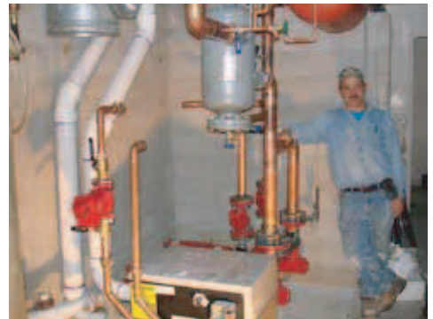
This pump in the mechanical room circulates glycol to the apartment units. The glycol comes through pipes from multiple geothermal wells in the well field, with each building having a separate well field.
