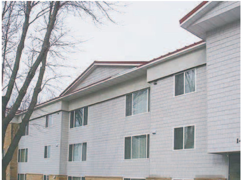
A view of the Hardishingle siding and the standing seam roof at Viking Terrace. Both materials work well in Minnesota's climate and are environmentally sound choices.
